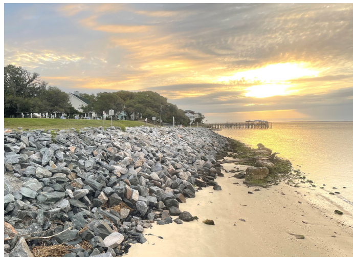
Hardened shoreline solution, rock revetment
