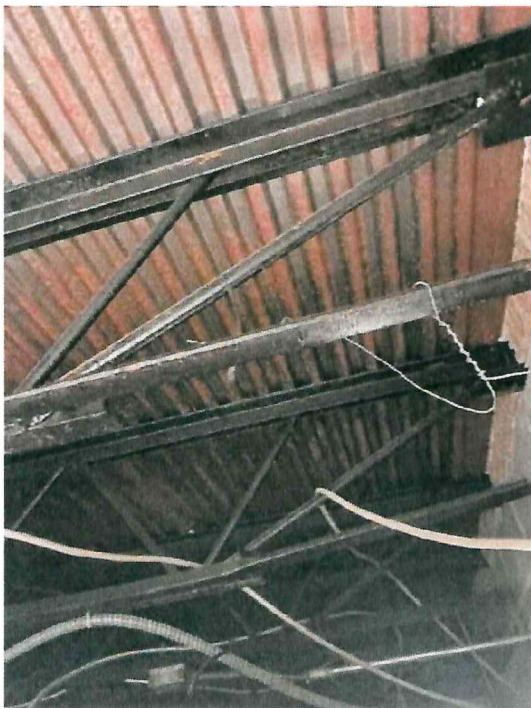
Metal Decking with Surface Corrosion
