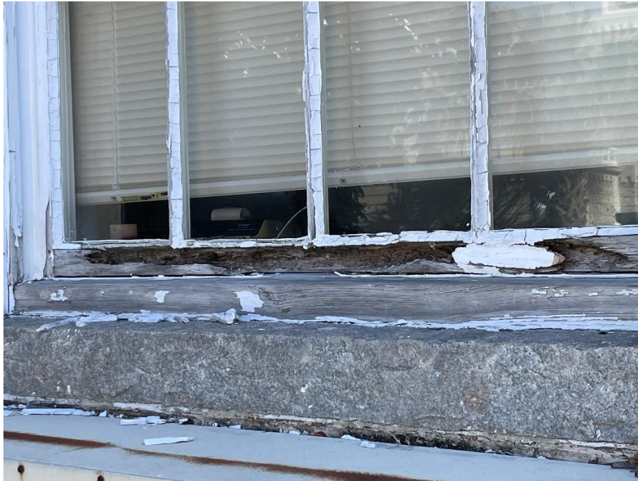
Photograph 3 – View of typical exterior window damage on the east side of the building of the original section.
