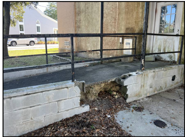
Damage and deterioration of foundation wall for the ADA concrete ramp
