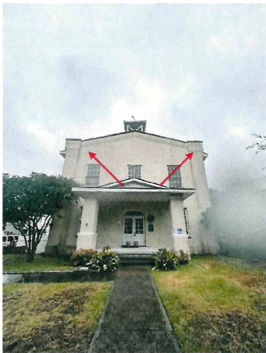
Southern Corbels and Walls of the Original Building Appear to be Experiencing Staining from High Concentrations of Moisture
