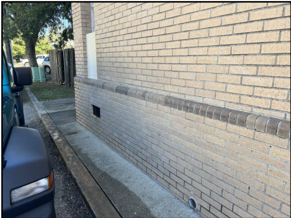
View of exterior indicating a crawl space type foundation
