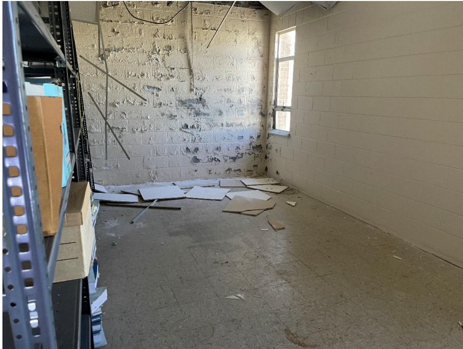
Photo 29 – View of room 203 with water damaged CMU walls.
