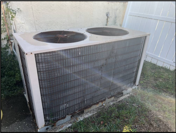
Luxaire 10-ton heat pump; manufactured in 1996
