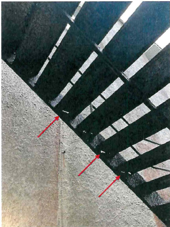
Northern Stair Stringers with Severe Corrosion – UNSAFE CONDITION
