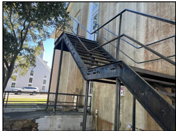
Overall view of the metal pole supported stairs that provides access to the 2nd story rear entrance
