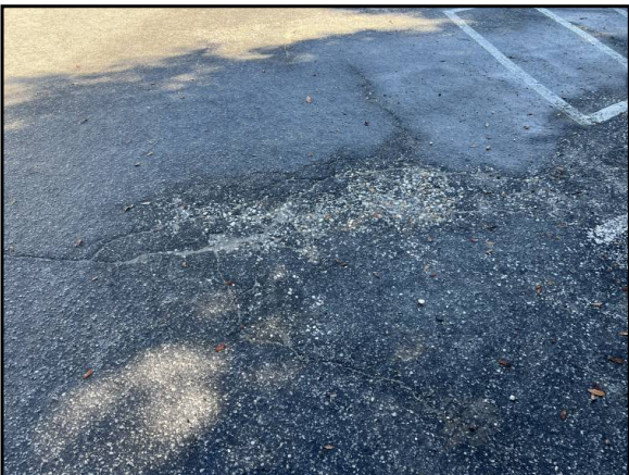
Deterioration of the asphalt paved parking area
