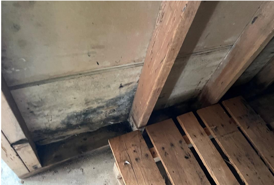
Photo 17 – View of the understairs closet by the bathroom with suspected mold growth on the gypsum lath.
