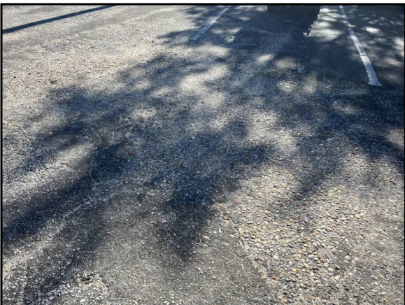
Deterioration of the asphalt paved parking area
