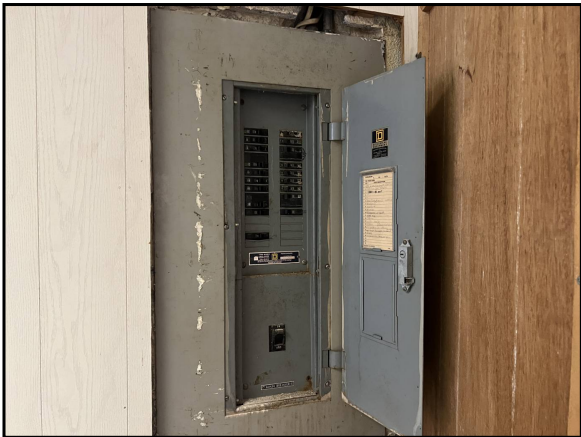
Typical condition of electrical panel box
