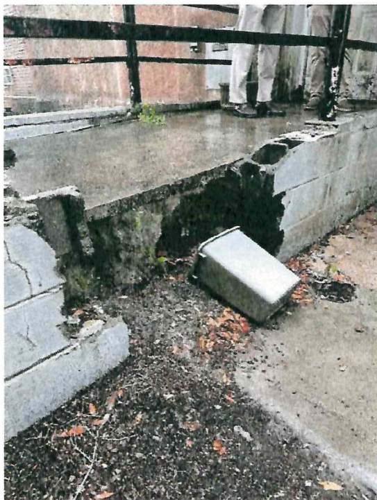
CMU Failure and Undermined Concrete Slab at West Side of North Exterior Ramp
