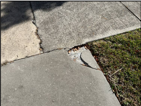
Cracked and deteriorated concrete walkway
