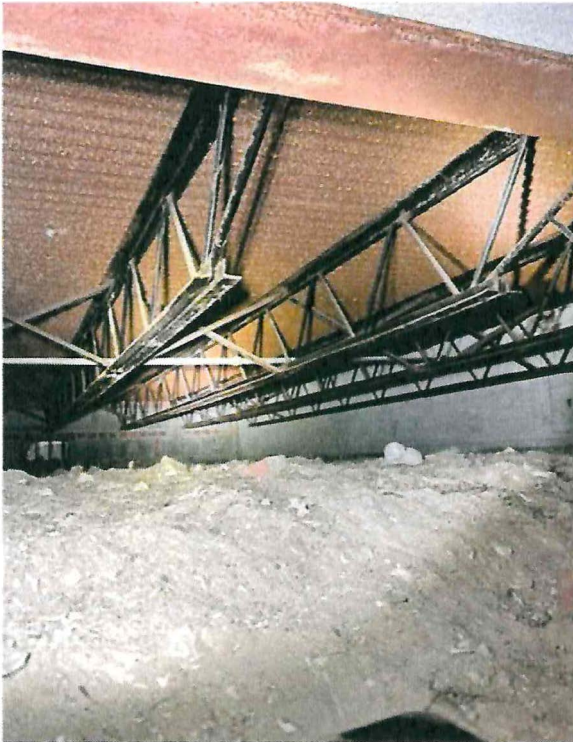
Joists and Metal Decking with Surface Corrosion
