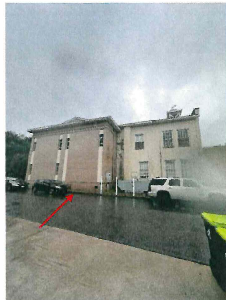
West Wing (Brick Veneer), Original Building with Cementitious Exterior Coating
