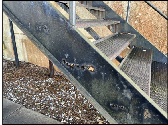
Closeup view of the rusted condition of the metal pole supported stairs
