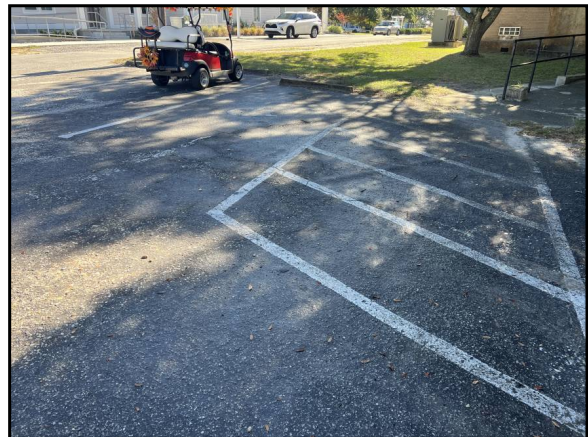
Faded parking stripping
