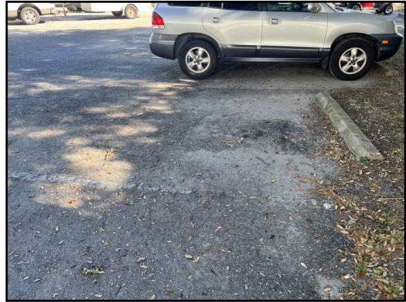
Deterioration of the asphalt paved parking area
