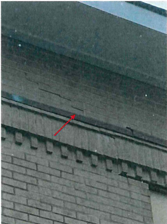
Stair Step Mortar Joint Crack
