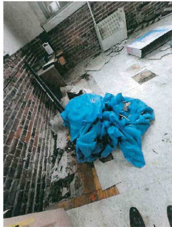
Southwest Corner of Original Building with Water Damage to Floor (Mechanical Room)
