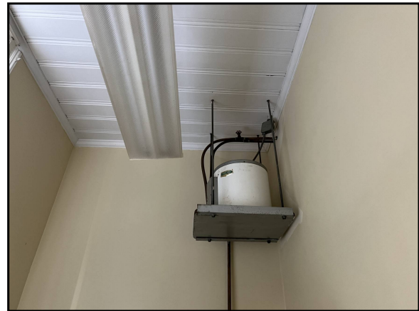
View of 30-gallon electrical water heater located in one of the bathrooms
