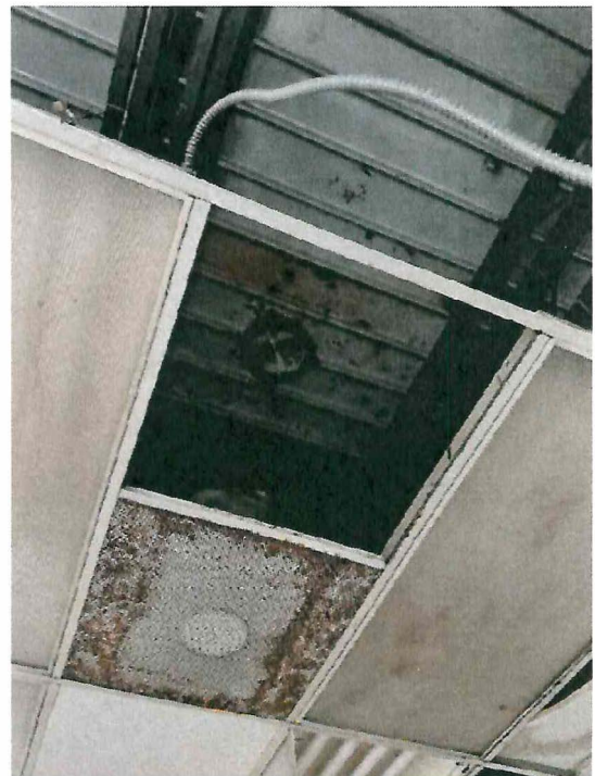
Filled Penetration in Metal Deck Above Second Floor
