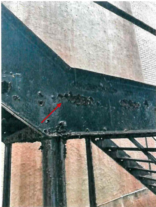
Northern Stair Entrance with Severe Corrosion and Deterioration – UNSAFE CONDITION
