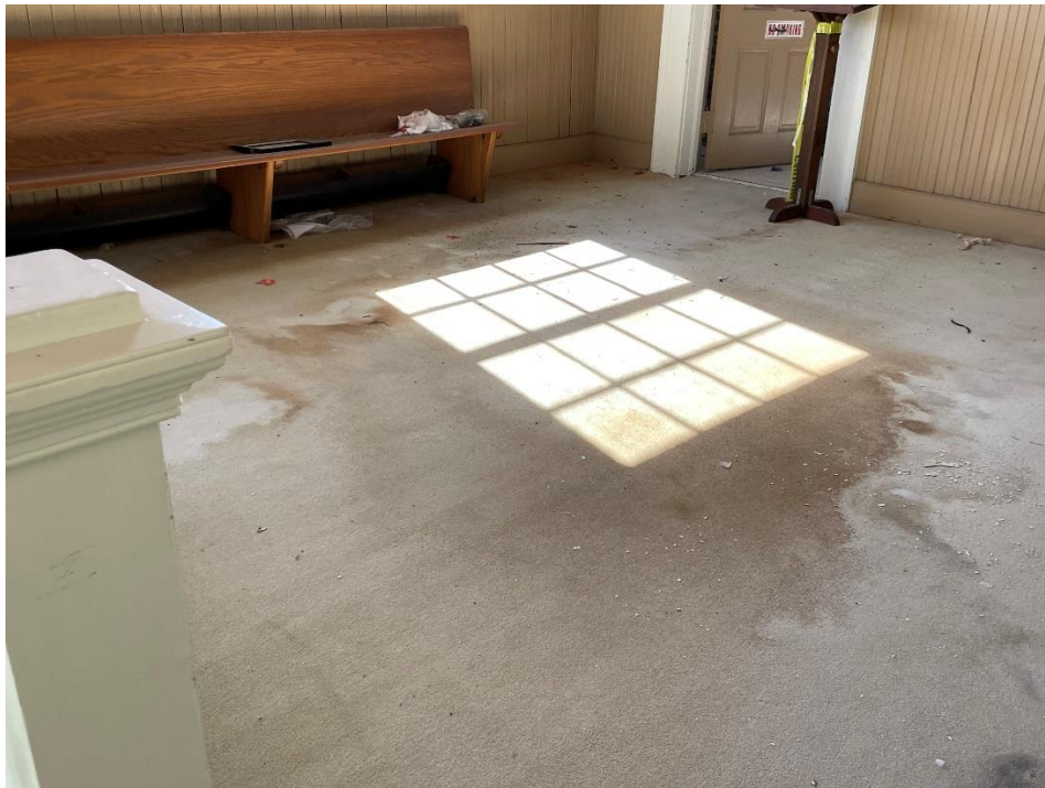
Photo 19 – View of water damage on floor on the second floor landing from a presumed roof leak.
