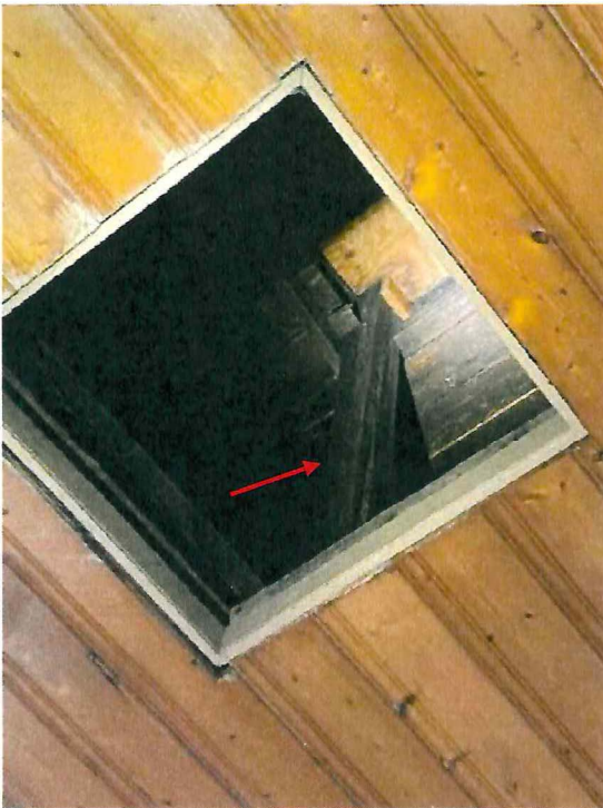
Timber Post Supporting Bell Tower (Active Water Leak Observed at all Four Posts at Roof Interface)
