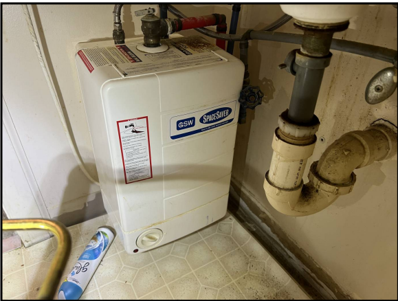
View of a on-demand electrical water heater located in one of the bathrooms
