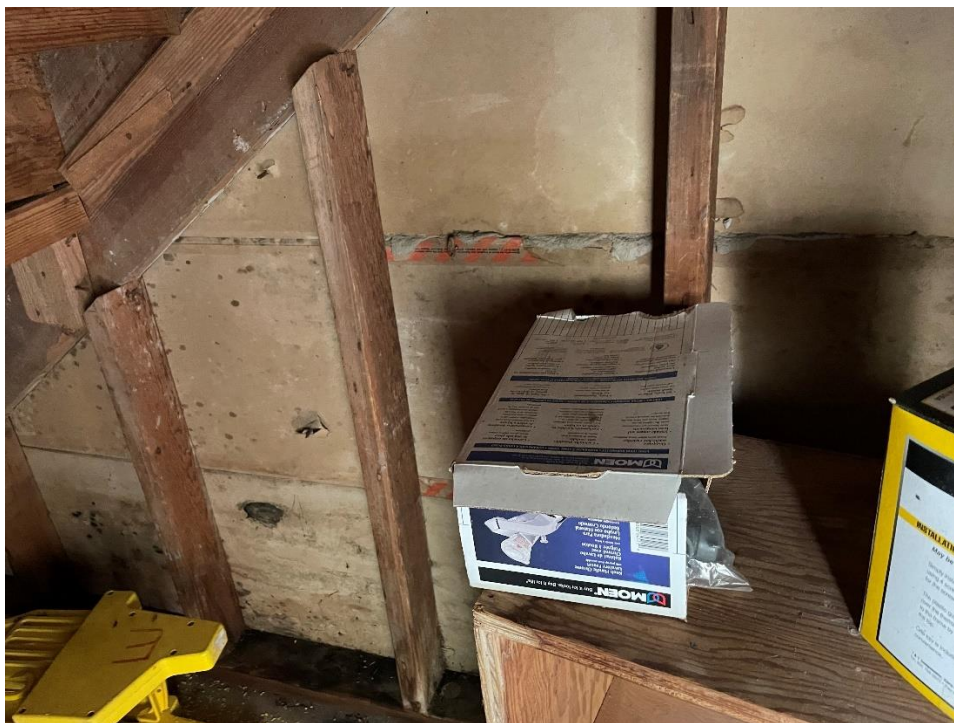
Photo 16 – View of the understairs closet by the bathroom with suspected mold growth on the gypsum lath.
