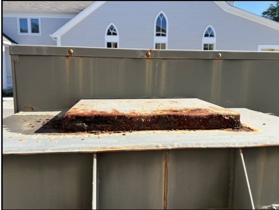
Observed rust atop the main electrical transformer
