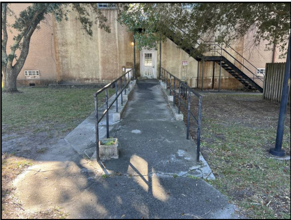
Concrete ADA ramp that provided access to the rear entrance
