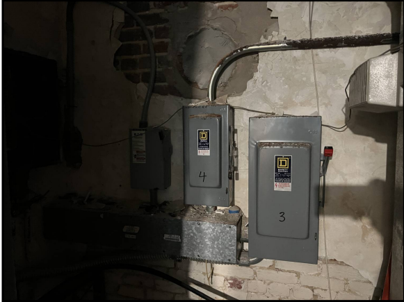
Electrical disconnects for some of the mechanical equipment
