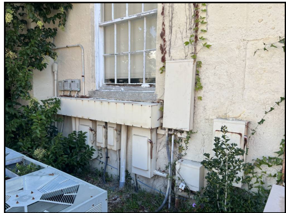
Electrical feeds and disconnects for the outside mechanical equipment
