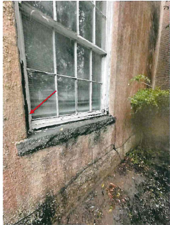
Typical Condition of Severely Deteriorated Wood Window Framing
