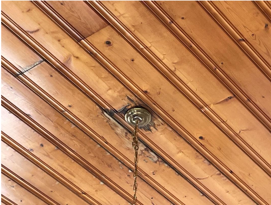
Photo 21 – View of water damage to the wood ceiling on the second floor landing. This ceiling is present throughout the first floor original section.
