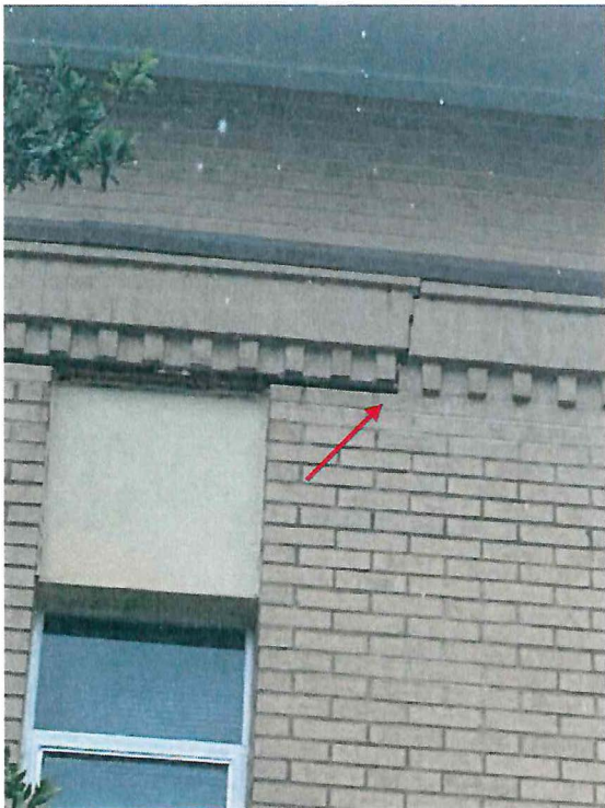
Advanced Lintel Corrosion and Joint Crack Above Window
