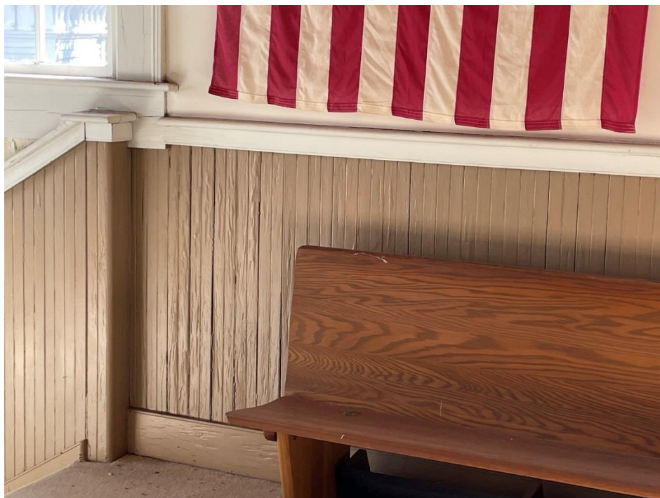
Photo 20 – View of water damage on wainscoting on the second floor landing.
