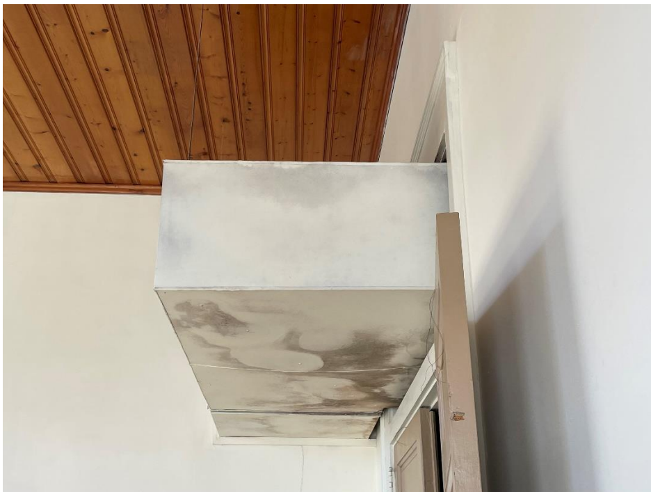
Photo 22 – View of suspected mold on the duct insulation leading into the courtroom.
