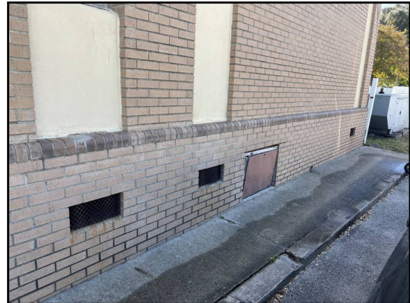
View of foundation vents and access door for the crawl space
