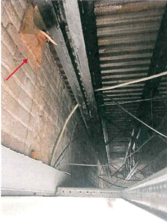
Steel Joist with Decking Above Suspended Ceiling, Plate with Threaded Rod for Assumed Building Cross Tie
