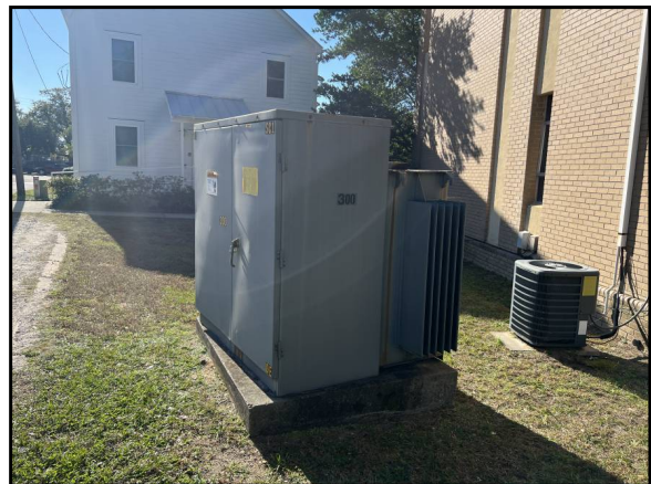
View of onsite electrical transformer
