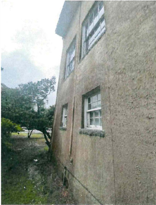
Eastern Wall Exhibiting Efflorescence
