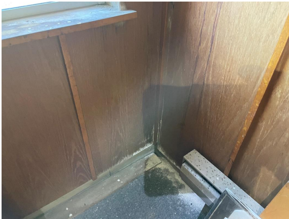
Photo 30 – View of room 207 with suspected mold on the wood paneling and carpet with evidence of CMU wall damage behind.
