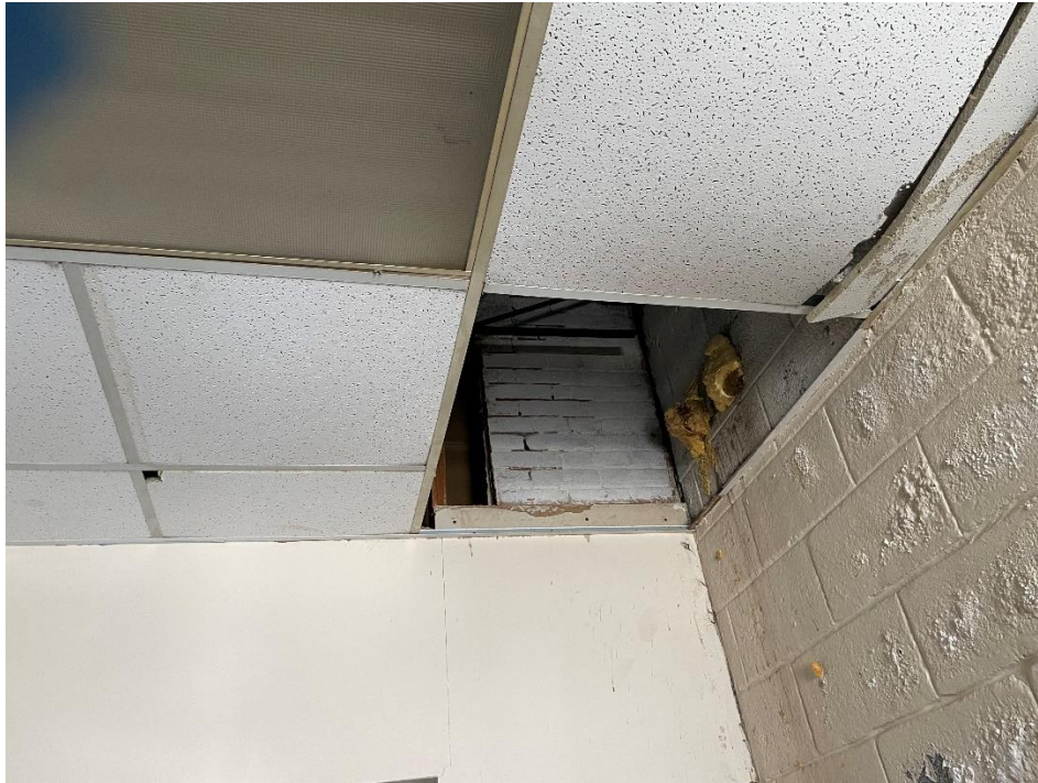
Photo 33 – View of the second floor back area joint of original building to east wing addition, area of suspected mold growth on the first floor.
