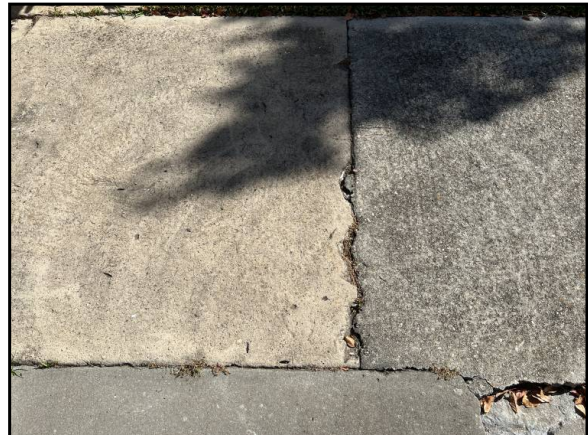
Cracked and deteriorated concrete walkway
