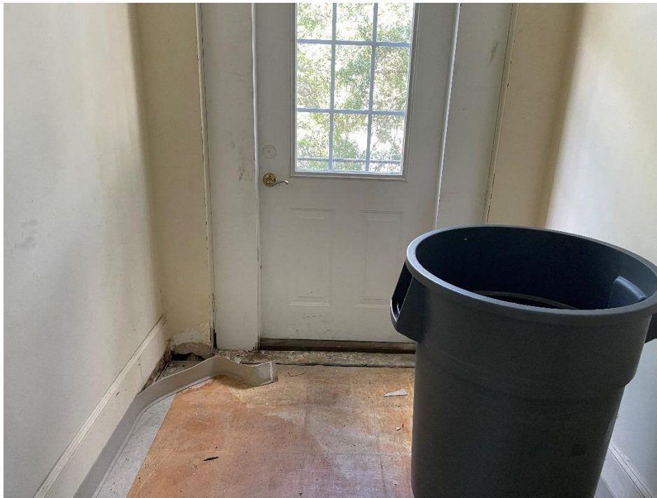
Photo 31 – View of the second floor back door with evidence of water damage around the base.
