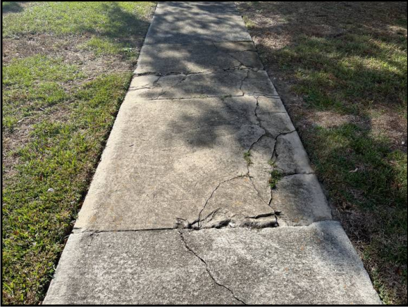
Cracked and deteriorated concrete walkway
