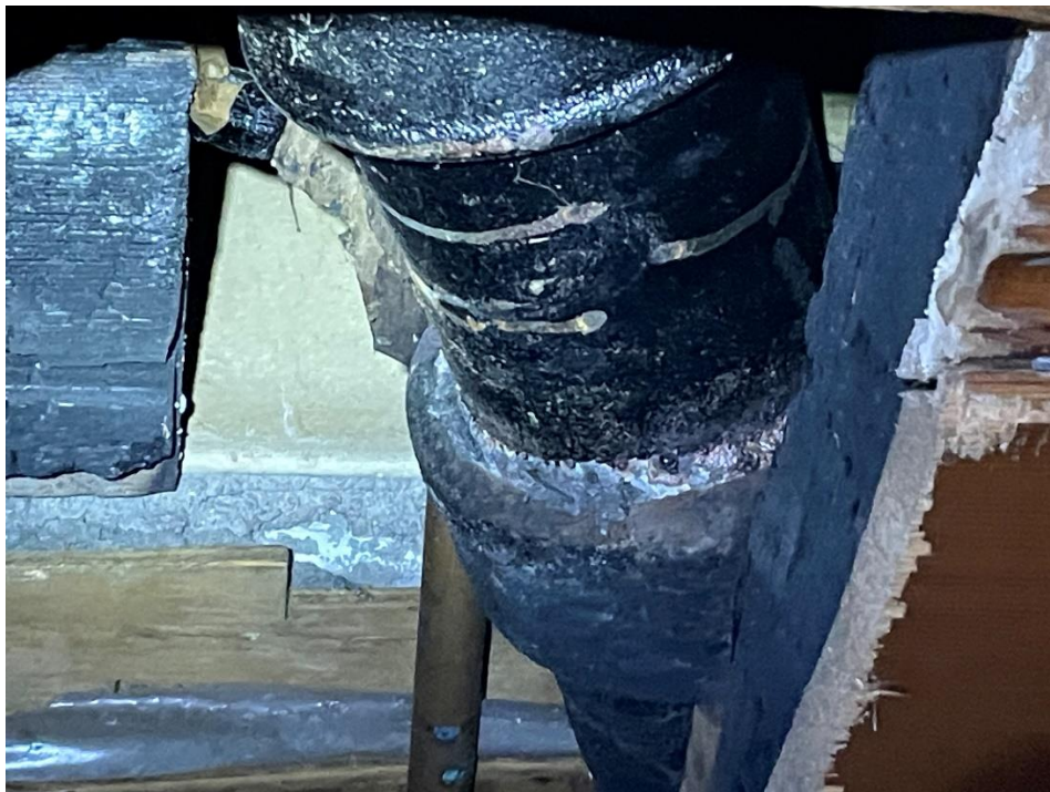
Photo 18 – View of the suspect ACM pipe insulation (black wrap) within the interstitial space between the first and second floor, above the wooden ceiling.
