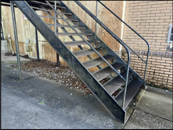
Observed rust at the metal pole supported stairs
