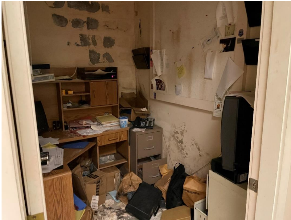
Photo 15 – View of the water damage and suspected mold growth in Room 15.
