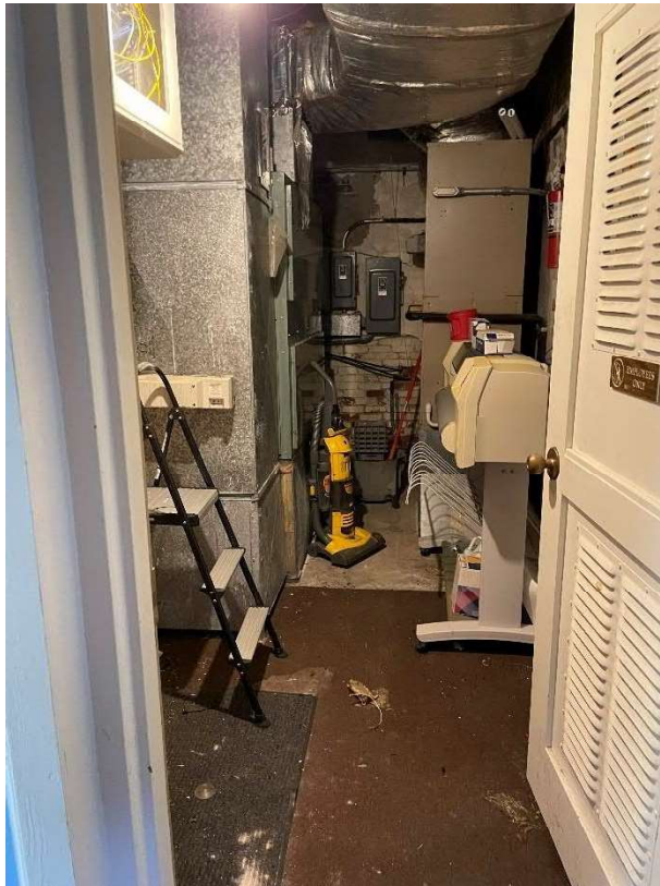
Photo 7 – View of the first floor mechanical room.
