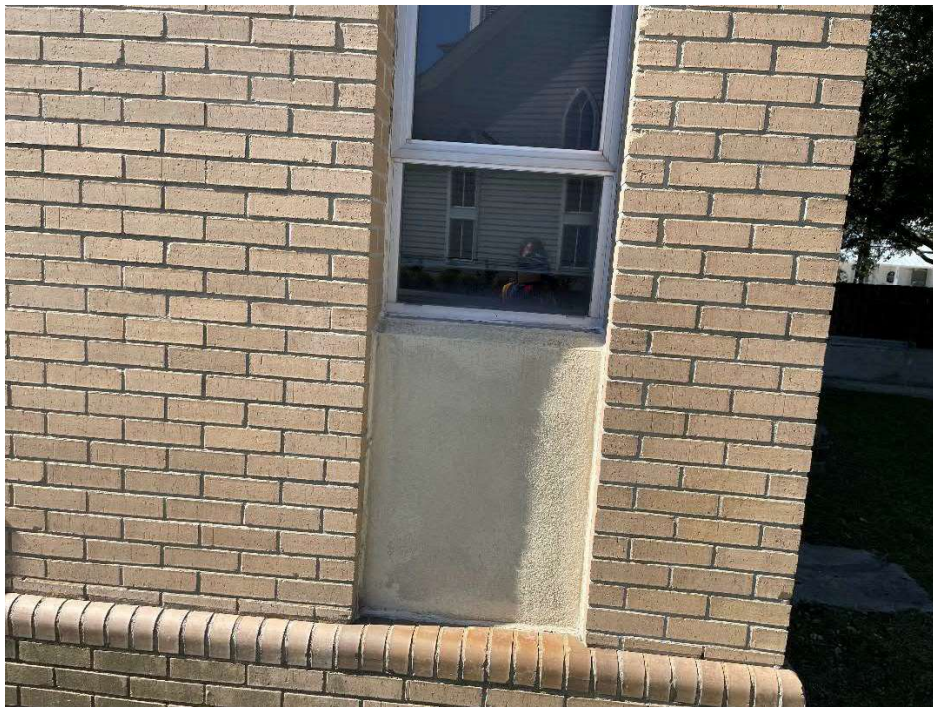
Photograph 4 – View of typical exterior on the east or west wing additions.
