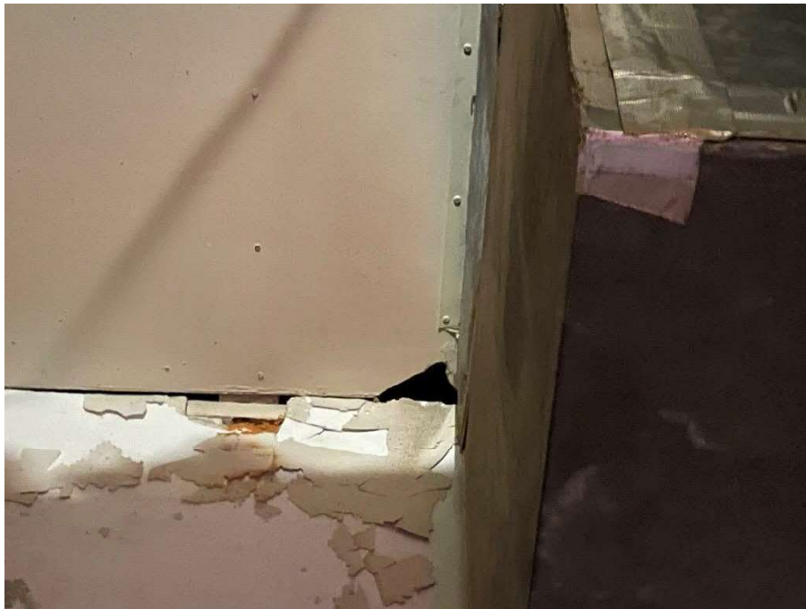
Photo 8 – View of suspect ACM cement board ceiling in the mechanical room.
