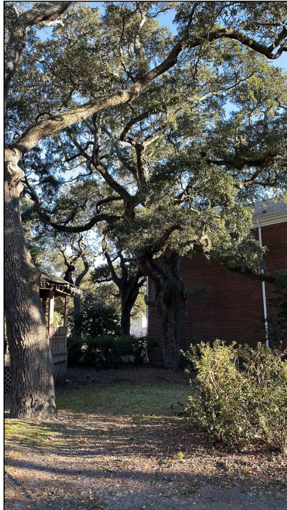
Photo 4: Looking east at live oak #8 showing the close proximity to the building.
