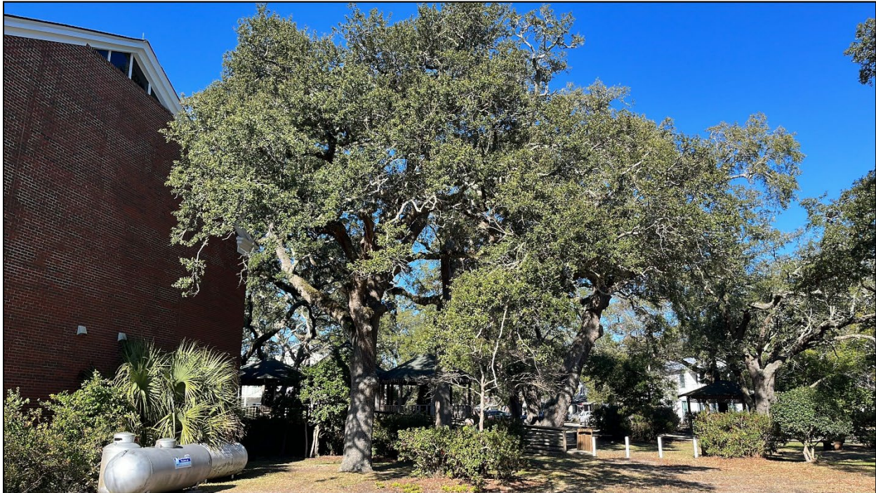
Photo 10: Looking north at live oak #22 showing the uneven crown and proximity to the building.
