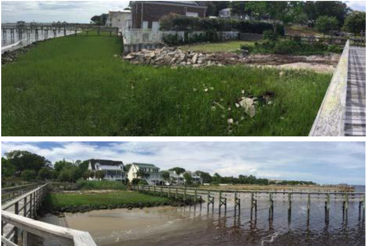
Figure 9: Photographs taken from the Kingsley Fishing Pier on 30 May 2018. Top – facing west showing the rock sill, marsh grass, vinyl wall, and protection along the park. Bottom – facing east showing the pier and the rock sill.
