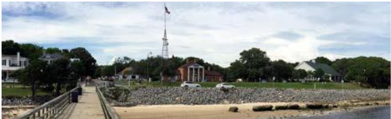
Figure 7: Panoramic view of the steep revetment abutting E. Bay St. with Oceanfront Park on the left and tabby stones in the foreground.
