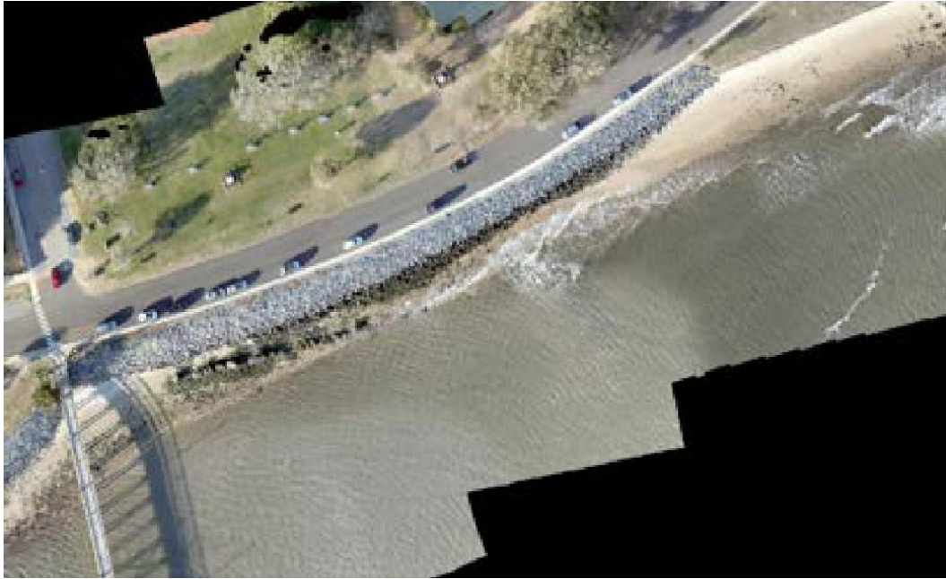
Figure 15. East section of the western area shoreline aerial image (courtesy of M&C).
