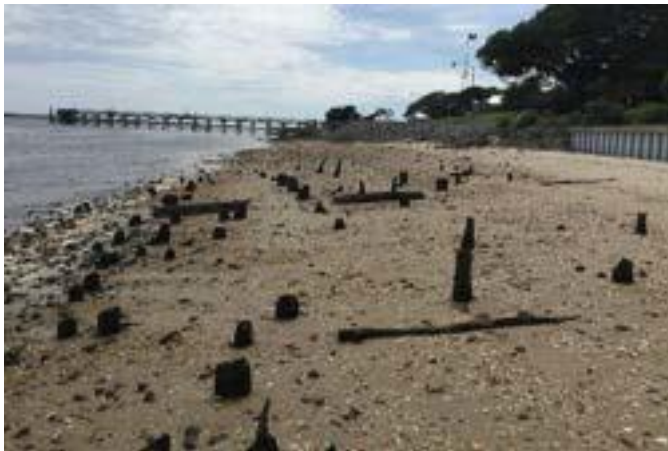
Figure 8: Photographs of the intertidal zone fronting the vinyl bulkhead.
