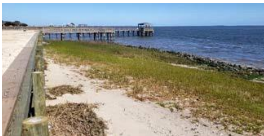
Figure 5. Eastern section of the shoreline illustrating bulkheads, Spartina and rock sill.
